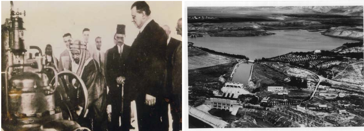
Figure 4. Left: The inauguration of the Palestine Electric Corporation's Naharayim power plant in 1933 by Emir Abdullah of Jordan. Its owner, Pinhas Rutenberg, looks on. Right: aerial photograph of the Naharayim power plant.
