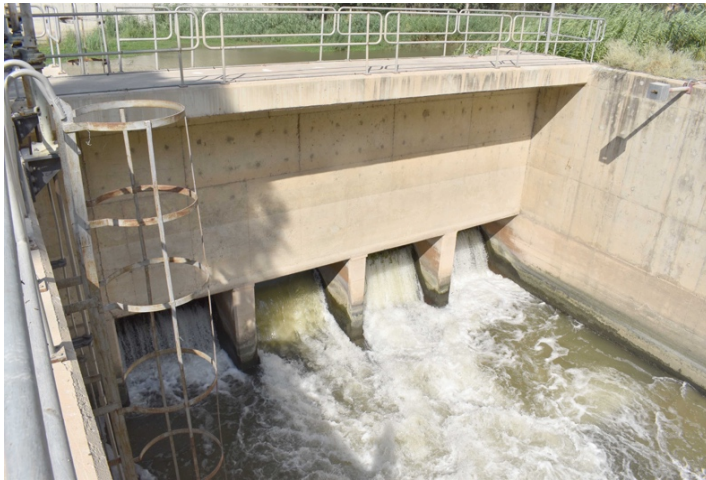
(c) The Adassiyeh Diversion Weir looking north.
