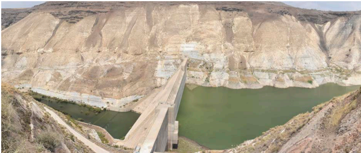
Figure 8. The Jordanian-Syrian Wehdeh Dam, September 2018, looking north, with Syria in the background and Jordan in the foreground.
